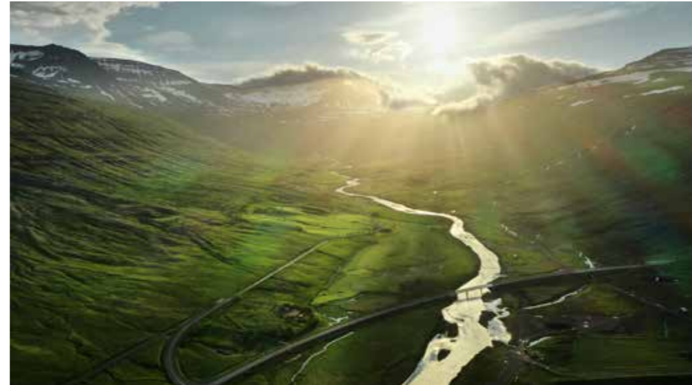
Tunnel mouth to the Norðfjörður tunnel at the bottom of Eskifjörður. Photo: Bjarki Jóhannsson
