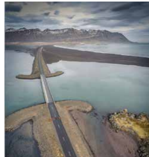
Bridge on road no. 1 close to Meleyri in Breiðdalur. Photo: Páll Guðmundur Ásgeirsson
