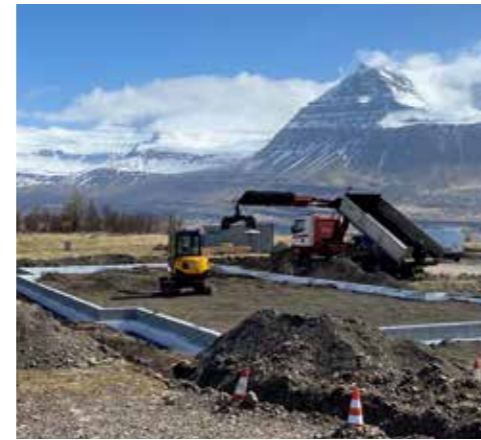
Construction project in Reyðarfjörður. Photo: Fjarðabyggð
